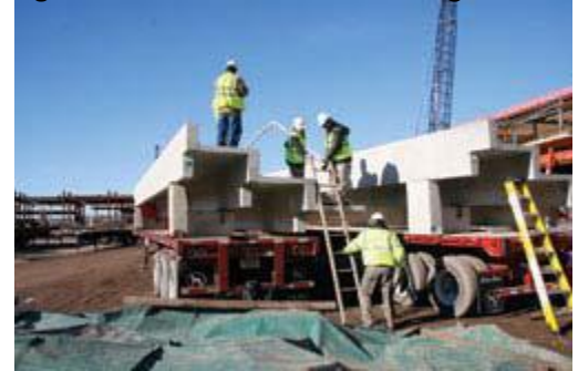
Figure 23: Precast Members Being Delivered
