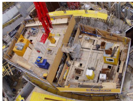
Figure 6: Super Climber Storage Area Courtesy of Doka
